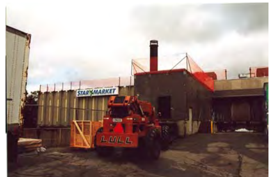
Custom debris containment at a re-roof project.
