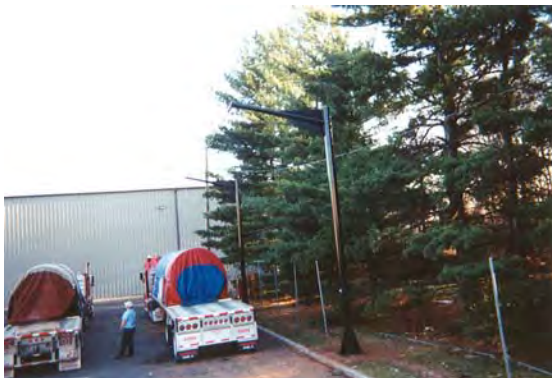
Outdoor Davit & Lifeline at a manufacturing facility.
